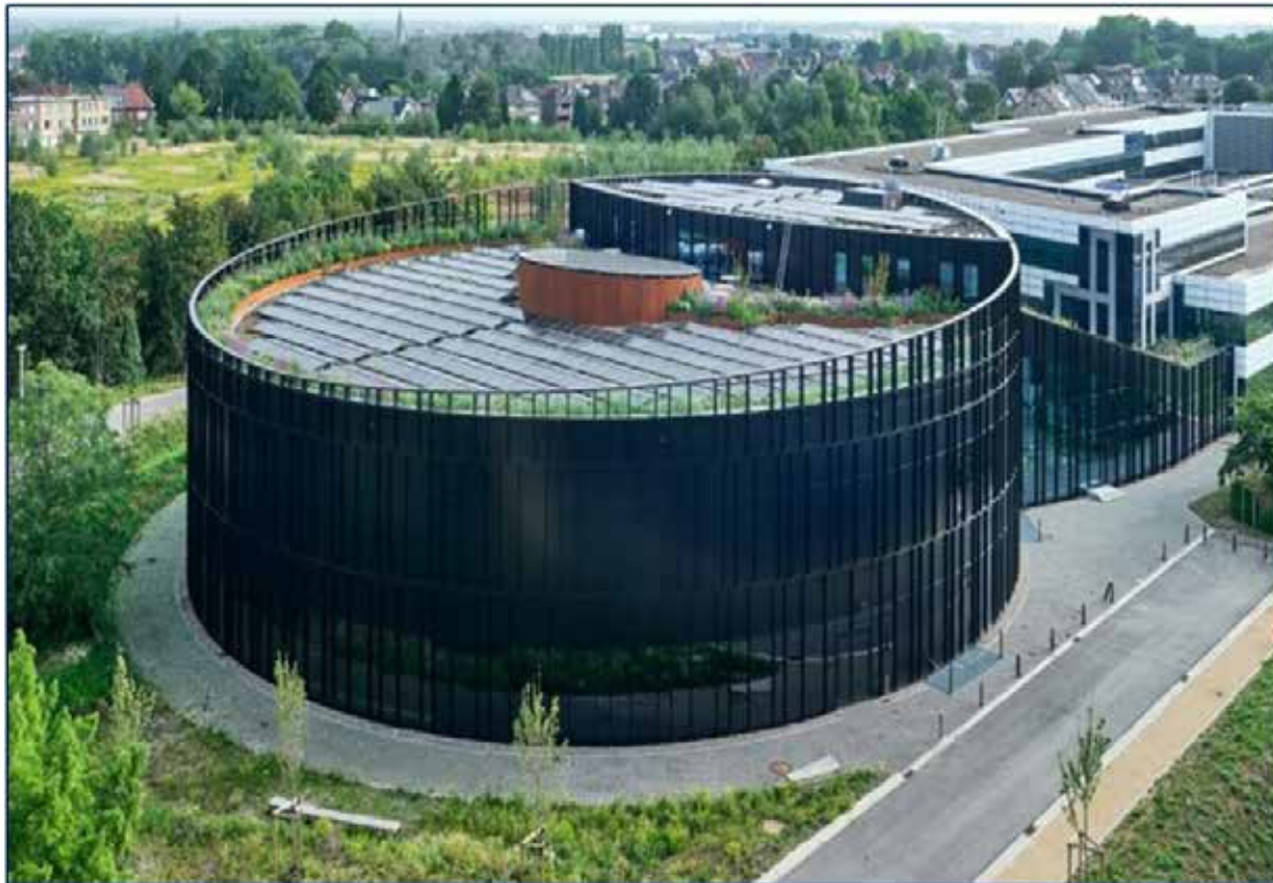
Figure 6: EUROCONTROL new Network Manager Operations Centre
