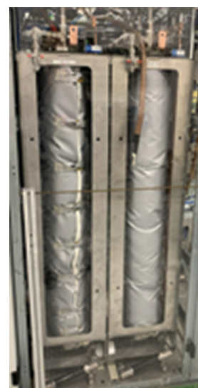
Figure 2d: two E-TAC reactors containing such stacks – Photo@H 2 Pro.
